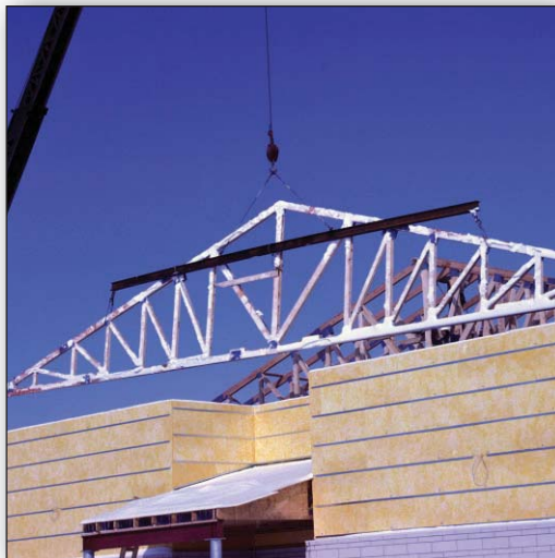
Erecting the trusses on the jobsite
