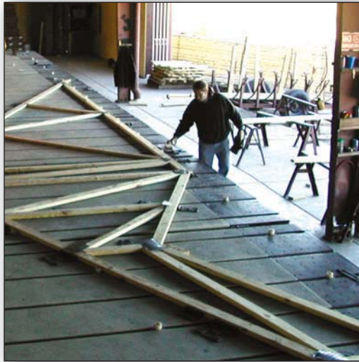
Manufacturing the trusses
