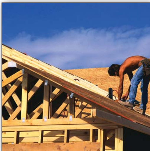
Permanent bracing system
